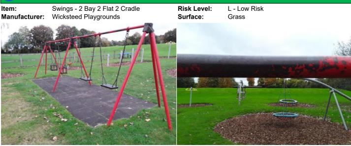
Finding: The paint is flaking off the metalwork
