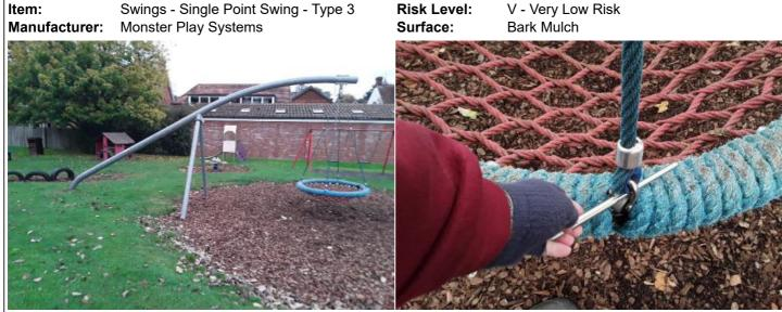
**Finding:** The connecting links are in excess of 8.6mm and less than 12mm and fail the requirements of BS EN 1176 Part 1; clause 4.2.13, Chains
