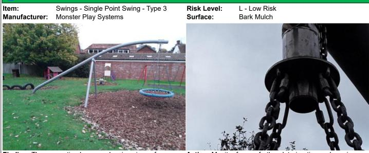
Finding: The connecting lugs are showing signs of wear
