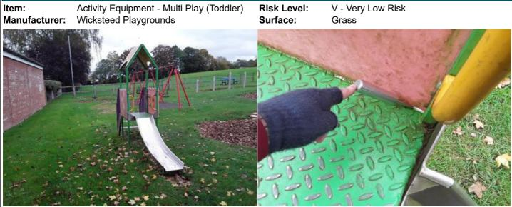
**Finding:** There is/are finger entrapment/s adjacent to the slide entry and the item fails to meet the requirements of BS EN 1176 Part 1 4.2.7.6 Entrapment of fingers
